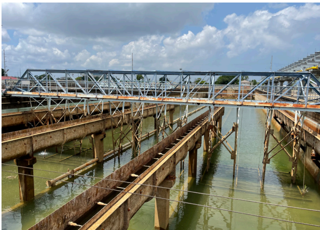
Settling Basin (offline for maintenance activities) at the Carrollton WTP.
